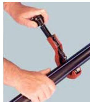
**Step 2** - Using a pipe scraper, scrape the end of the pipe equivalent to the depth of the socket, plus at least 10% for safety margin. Removal of the smooth, oxidized layer on the surface of the pipe is imperative to obtain a good fusion joint. Once prepared it is very important not to handle this area or allow it to get dirty.
