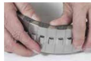
If the pipe is under 75mm pay extra attention to the ends of the strip to ensure they have been shaped correctly. Push one of the prongs of a bracket through the notch at one end of the strip. Fold the strip around the pipe and push the other prong through the notch on the other end of the strip. The bracket can be gently hammered in to position if pushing is difficult. Attach the bracket to the wall or floor as described over and shown on the box drawings. Fix the other bracket(s) as required.
