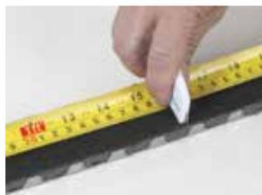
Cut through the Graftex at the appropriate position eg. for a 114mm OD pipe, cut at segment marked 30.
