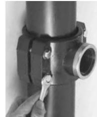
**3. Use a spanner to tighten bolt heads making sure not to over-torque.**
