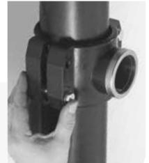
**2. Taking care to seat gasket in the branch outlet, bolt both halves together.**
