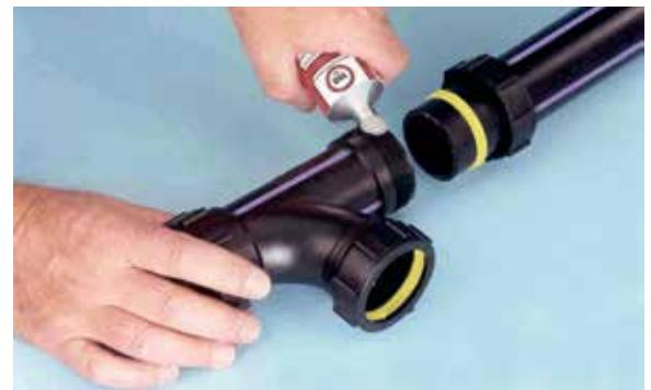
Loosely assemble the joint and proceed to hand tighten each nut. Using two Vulcathene spanners. The joint should then be tightened further to its full thread capacity.
