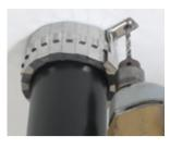
20mm x 5mm steel anchors provided, through the holes in the brackets provided.
